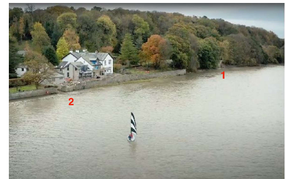
Photo, showing ramp (1), nearest road (2)
