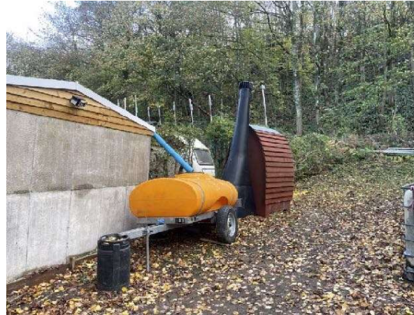
Water & Drainage. Rainwater currently only source of water. This may present significant H&S risk to the club going forward
